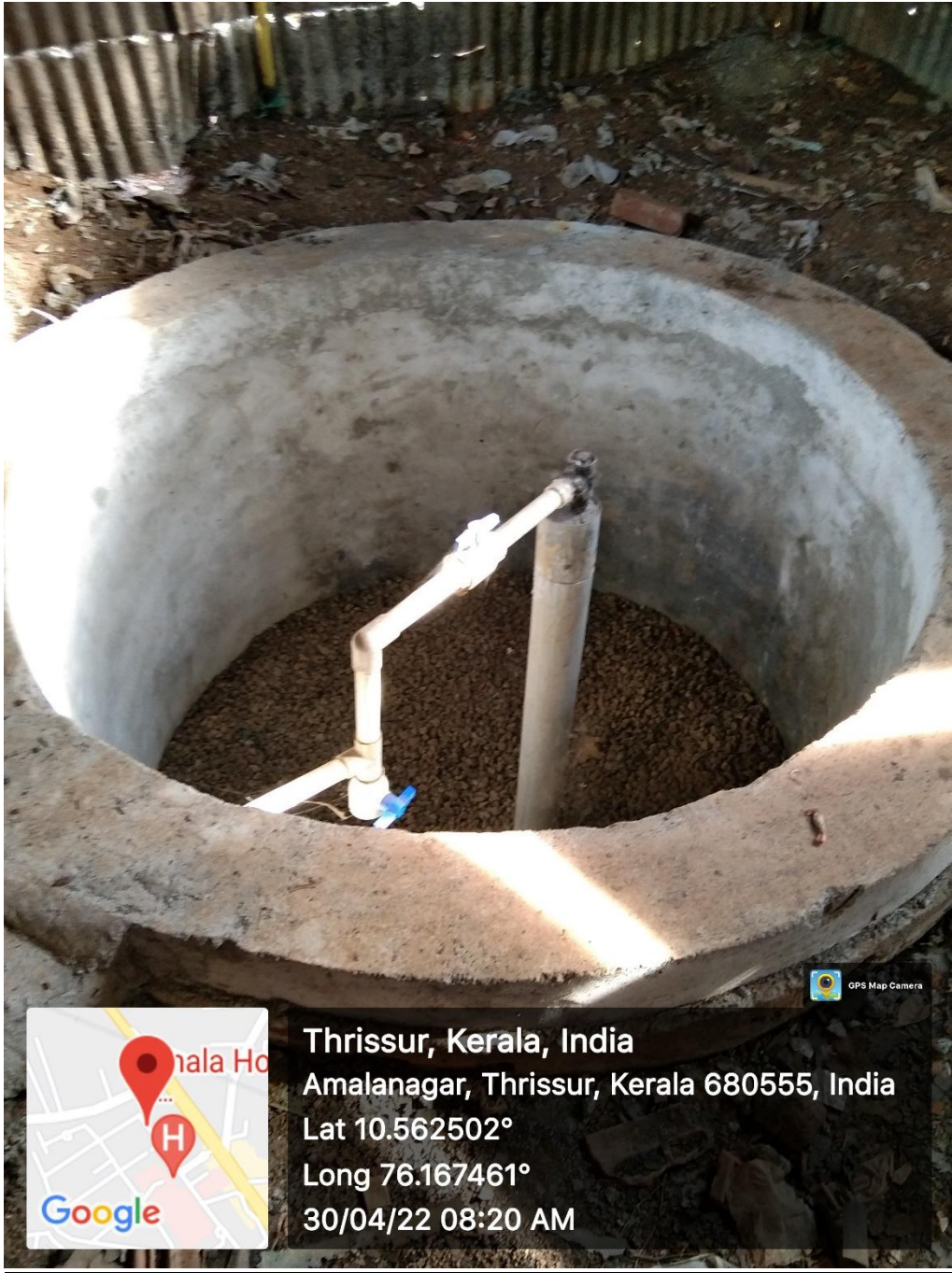
ACON, BIOGAS PLANT FOR DISPOSING FOOD AND GARDEN WASTE, NEAR TO THE LEFT SIDE OF THE COLLEGE BUILDING
