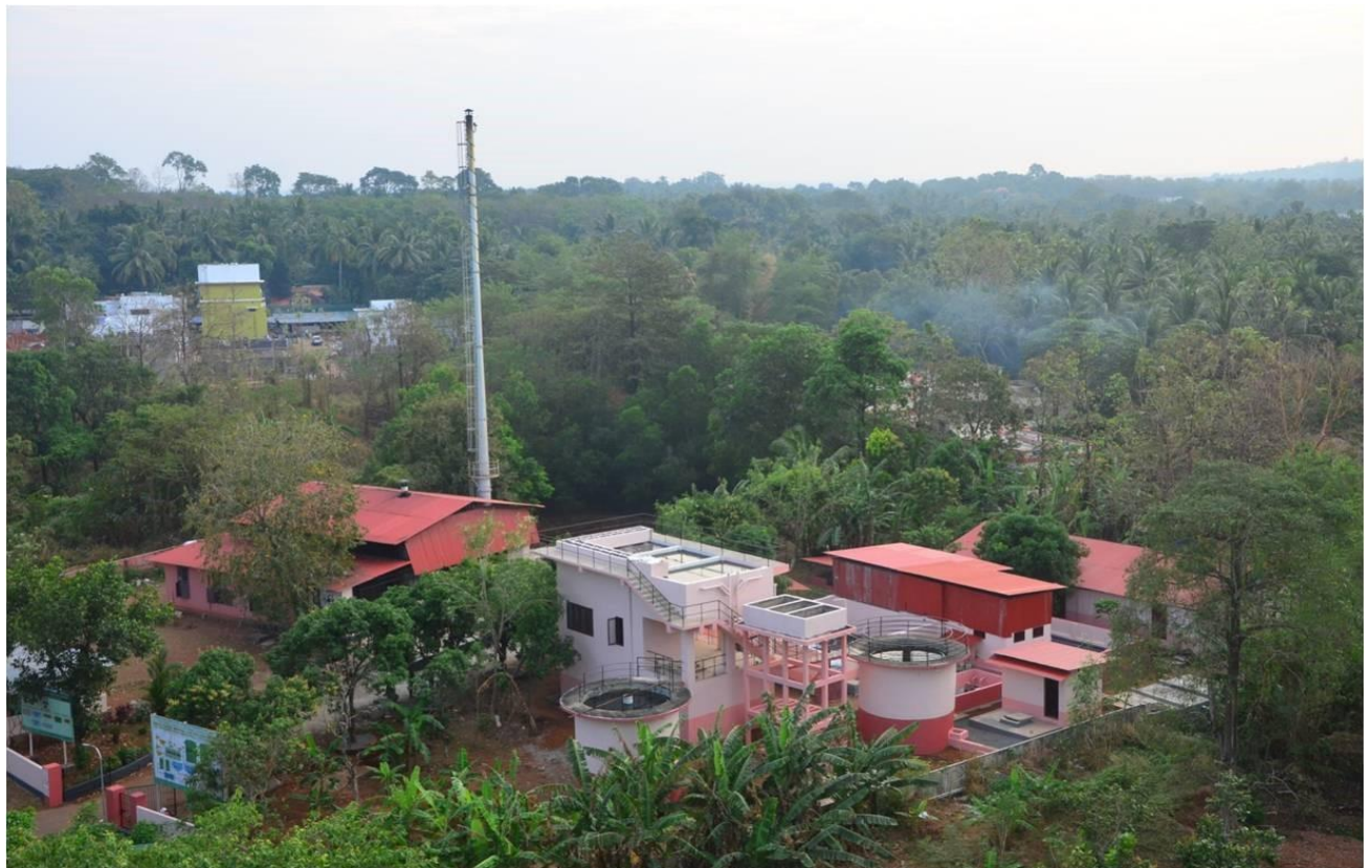
ACON, WASTE WATER RECYCLING PLANT
